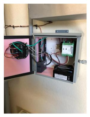
The typical voltage monitoring installation at CPEC consists of a Shark® 200 meter with a V3 switch and a Sierra Wireless RV50 4G cellular router, with UPS to provide meter power and communication capability during outages (See photo on the left).
